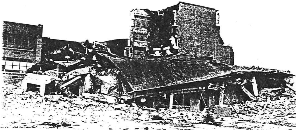
New Helena High School after the shock of October 31, 1935, which caused the total collapse of the north wing
