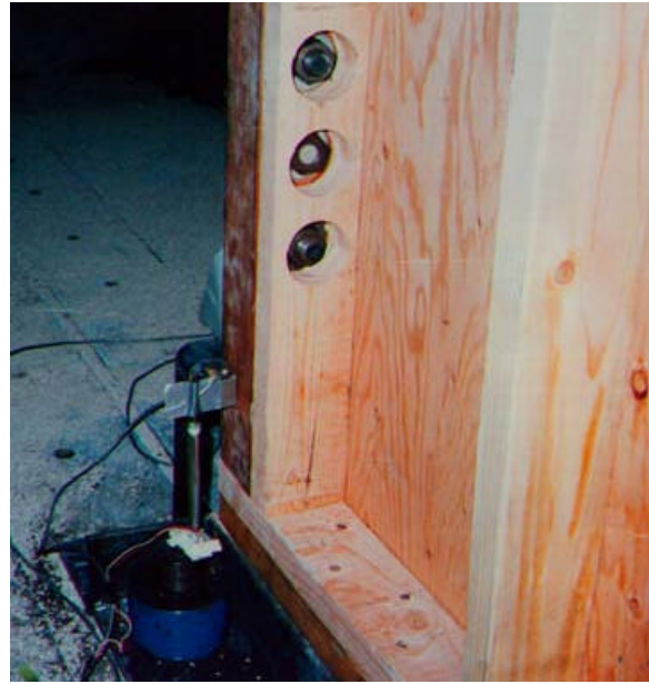
Figure 6, Sill nailing, hold down installation and vertical deflectometer
