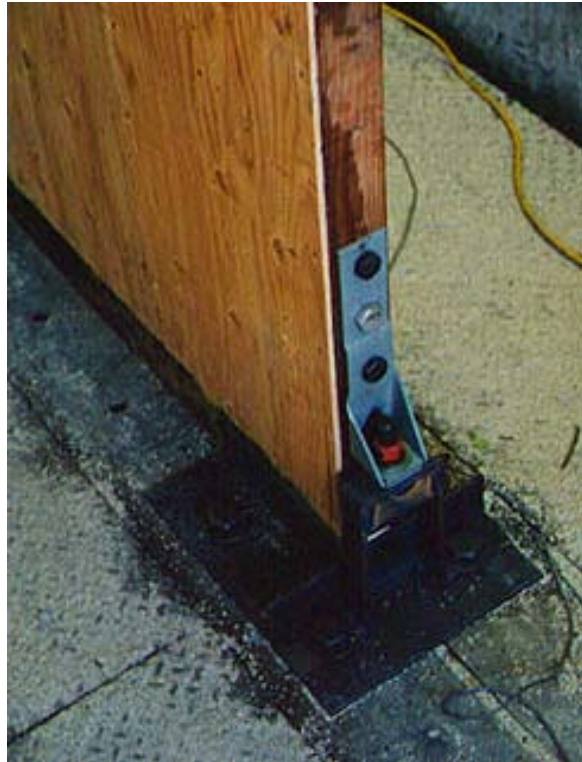
Figure 4, Base restraint and hold down
